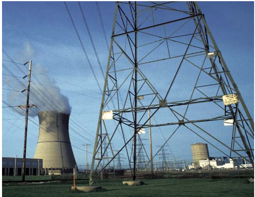
Outside the Davis-Besse nuclear power plant.
